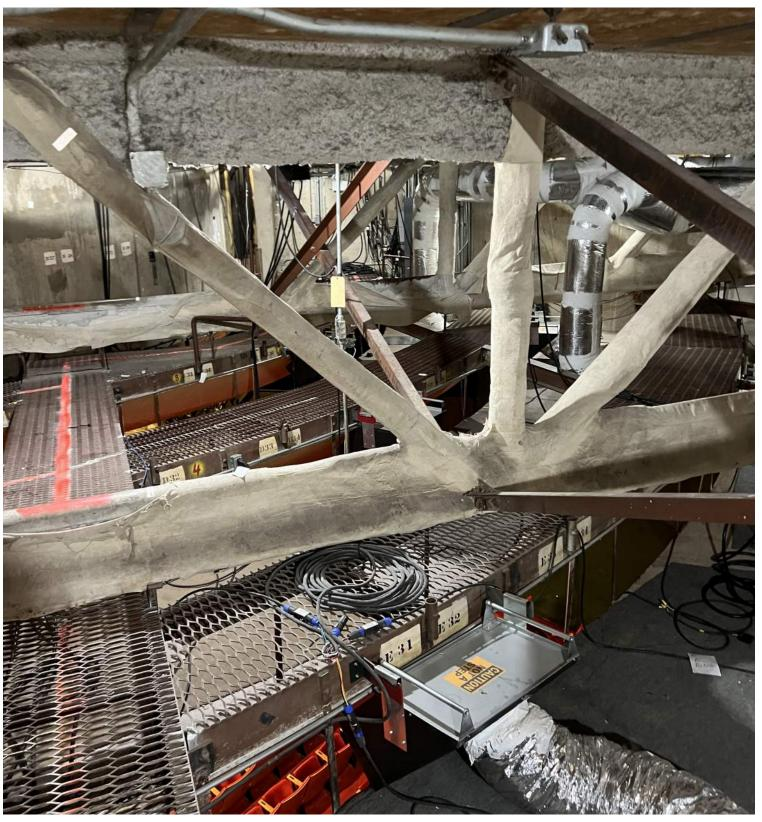
**Image 29** Existing attic condition. Roof trusses are fireproofed.
