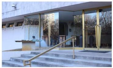
The non-original south entry paving, handrails, and fountain are in fair to poor condition.
