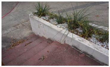
Concrete retaining walls are in fair condition with failing paint and areas of delaminiated concrete.
