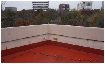
Built up roofing on terraces in fair to poor condition.
