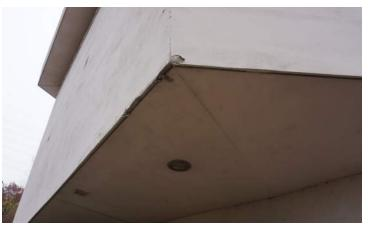
Delaminated coatings and deteriorated concrete is typical at overhang edges. Exterior lighting and mechanical vents in soffits in fair condition.
