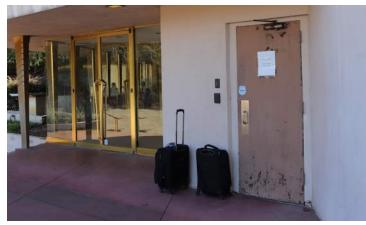
Exterior hollow metal doors are in fair condition with failed paint.
