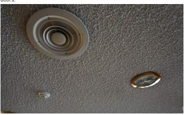
Circular flush-mount lense lighting typical of the building seen at right. MEP and life safety devices are randomly placed across lobby ceiling.
