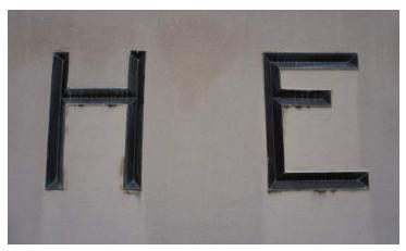
Bronze lettering on the building sign is in good condition, though is causing some soiling to the surrounding concrete.
