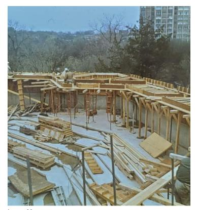
Image 22 Construction of the house balcony and installation of roof trusses
