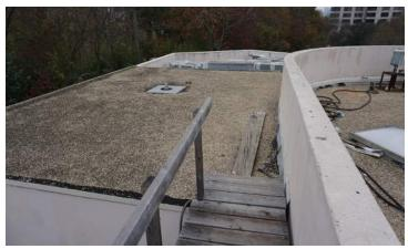
Flat roofing is at the end of its serviceable life.
