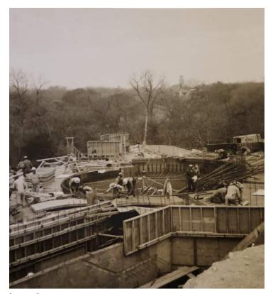
Image 4 Construction of original dropped floor stage, courtesy of DTC Theater Archives
