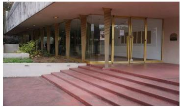
Exterior red-stained concrete steps are in poor condition.
