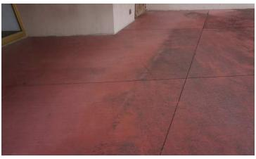
Exterior red-stained concrete pavers are soiled, cracked, and previously repaired.
